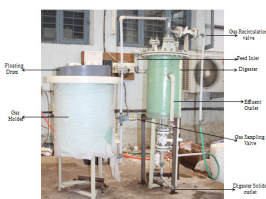
Figure 3: Bio gas generation from food waste
